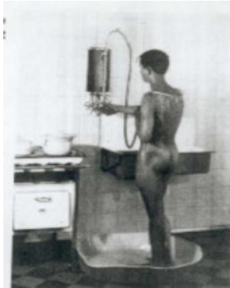
This combination was developed for flats without a bathroom in 1928 and it enabled a large part of the population the use of this wall-thermal for their personal hygiene.
