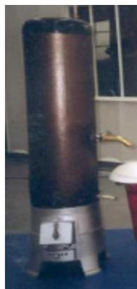
The first Junkers' standing coal-burning bath water heater worked on the principle of a hydraulic heater with an extended heating surface.
